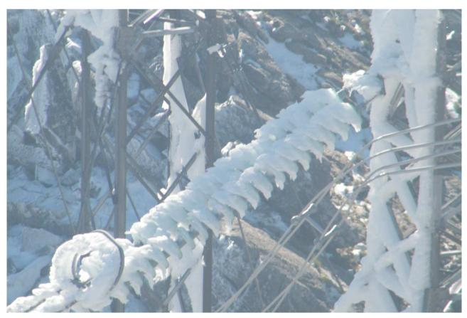
Figure 4: Picture showing the snow build up on the existing Droerivier – Proteus 400 kV line
