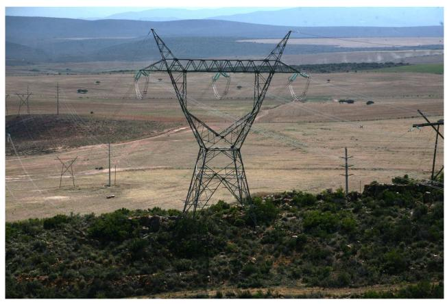
Figure 5: Picture showing 2 Dx lines running parallel to Droerivier Proteus 400 kV line
